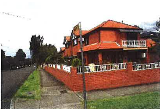
Photo 16: Corner of Stanley Street and Mitchell Road.
